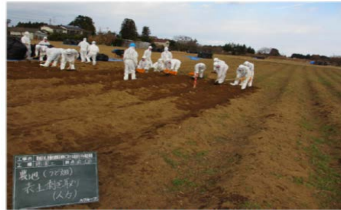
Manual topsoil stripping
