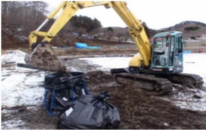
Topsoil stripping (mechanical digger)
