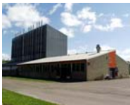
Waste Treatment Plant
