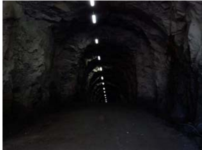
Entrance tunnel August 2007
