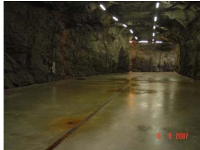
Storage tunnel August 2007
